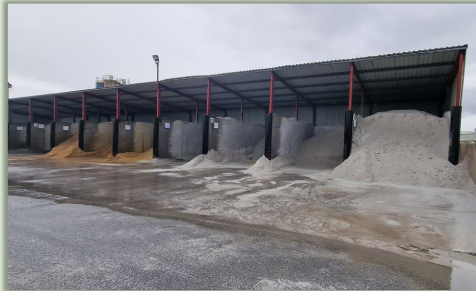
Segregation and labelling of aggregates is important
